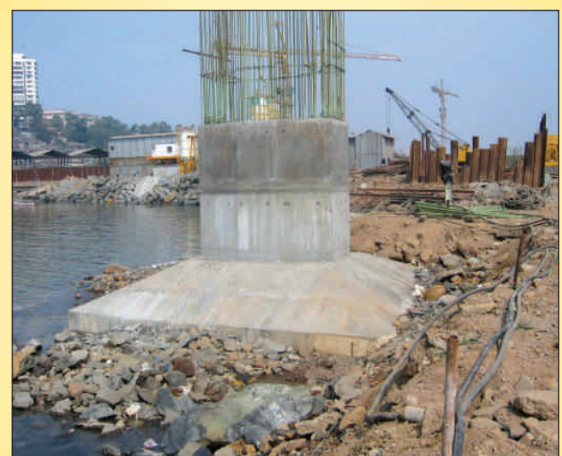
▲ Sea by-pass pier footing using fly ash based concrete in Mumbai
