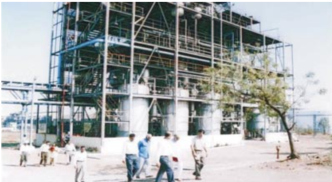
Ethyl Lactate from Molasses Project Under Commissioning at Godavari Sugar Mills Samirwadi, Karnataka
