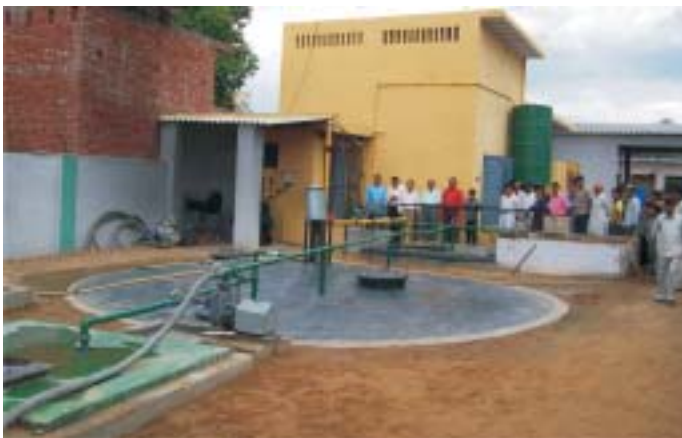
Model Milk Collection Parlor at Bharna run by biogas plant (2TPD capacity)
